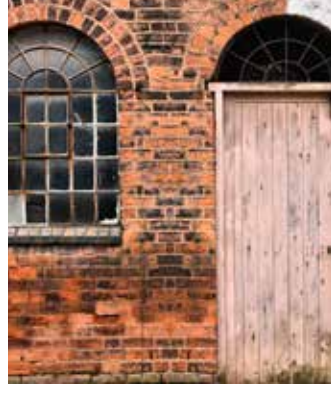
ARCHED WINDOW AND DOOR
