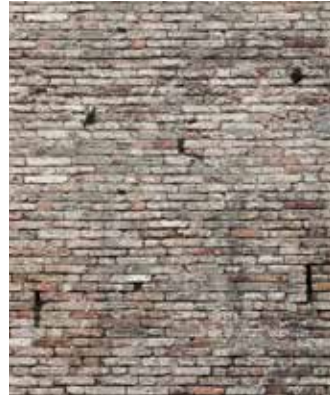
OLD GRUNGY BRICK WALL
