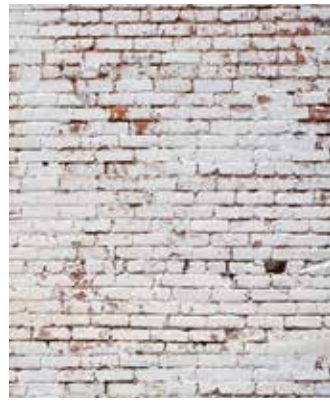
WHITE PAINTED BRICK WALL
