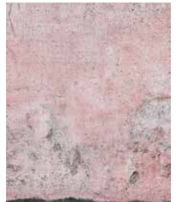
PLASTER WALL PINK
