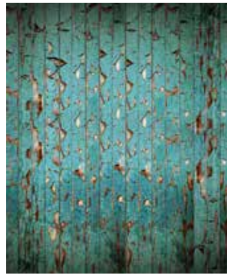
PEELING PAINT TEAL
