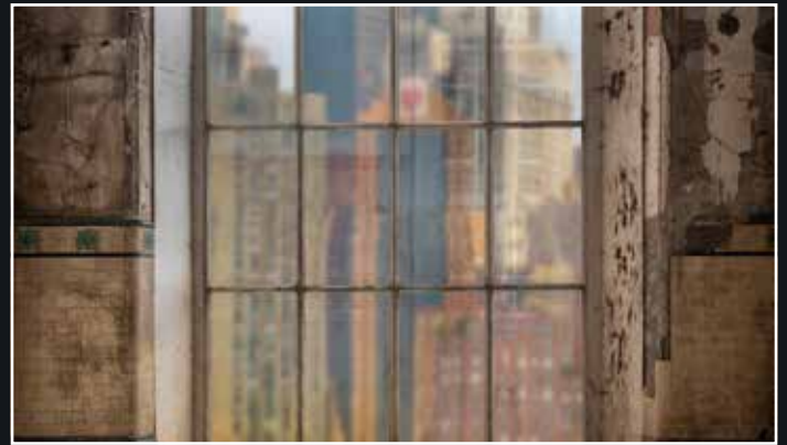
DERELICT TILED WINDOW NY
