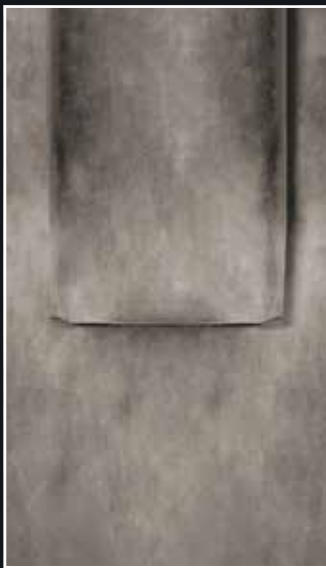
CONCRETE CENTRE STACK
