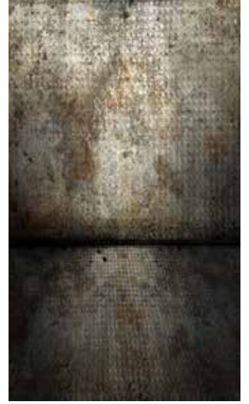
METALLIC RUST WALL
