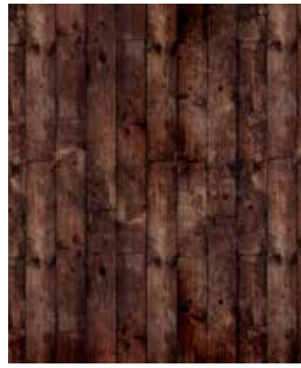
FLOOR WOOD STAINED BLACK
